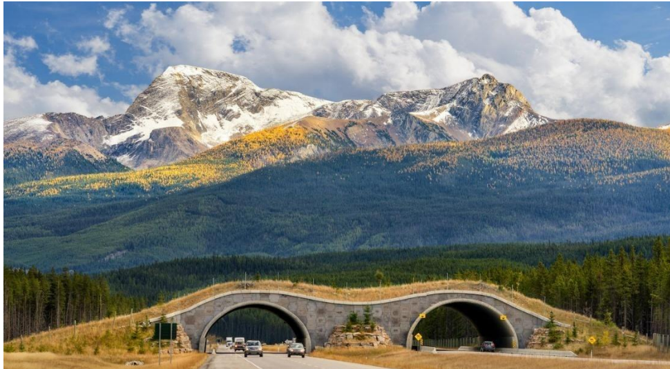
FIGURE 3- Banff Wildlife Overpass in Canada
